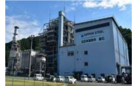
Thermal power plant in North Nippon Works, Kamaishi Area (output: 149,000 kW)
