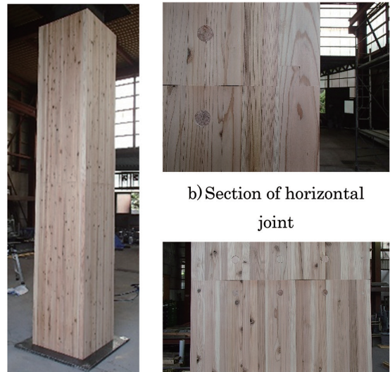
a) Full view of mockup b) Section of horizontal joint c) Front view of horizontal joint · wooden plug
