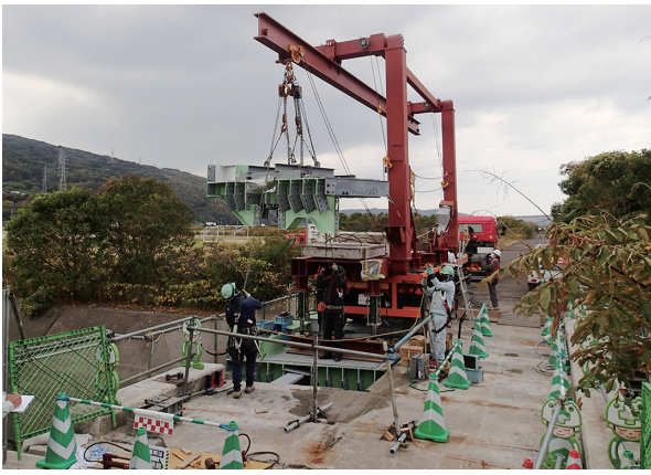
図 11 施工状況 Midorikawa bridge under deck replacement work
