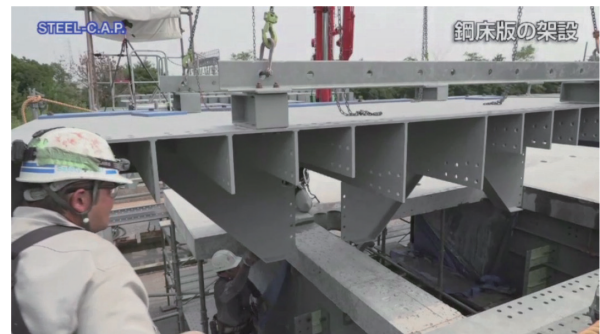
図 3 架設状況 Panel erection in mock-up test
