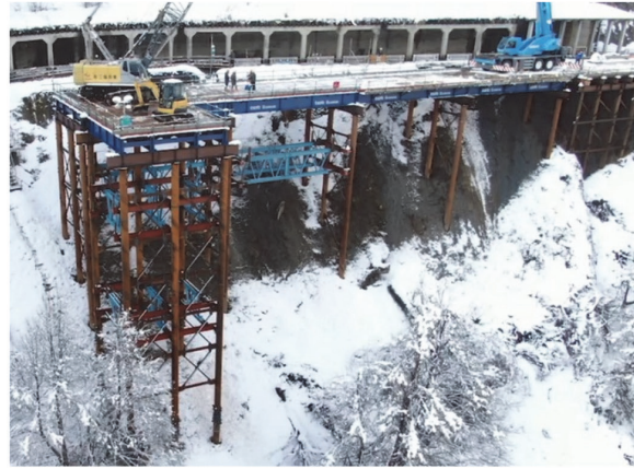
(b) Example using steel pipe piles
