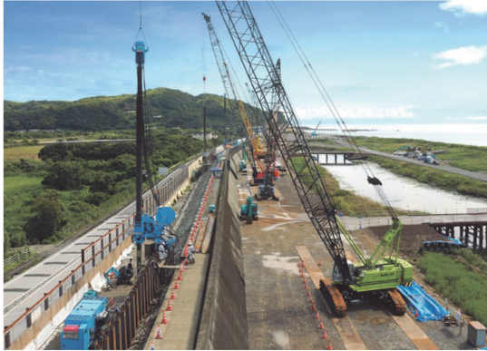
(a) Double steel sheet pile walls constructed using Press-in Method
