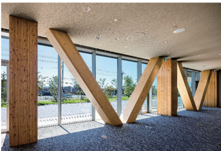
図9 木鉄ハイブリッド耐火柱 (適用例) Application of wood-steel hybrid fire-resistant column
